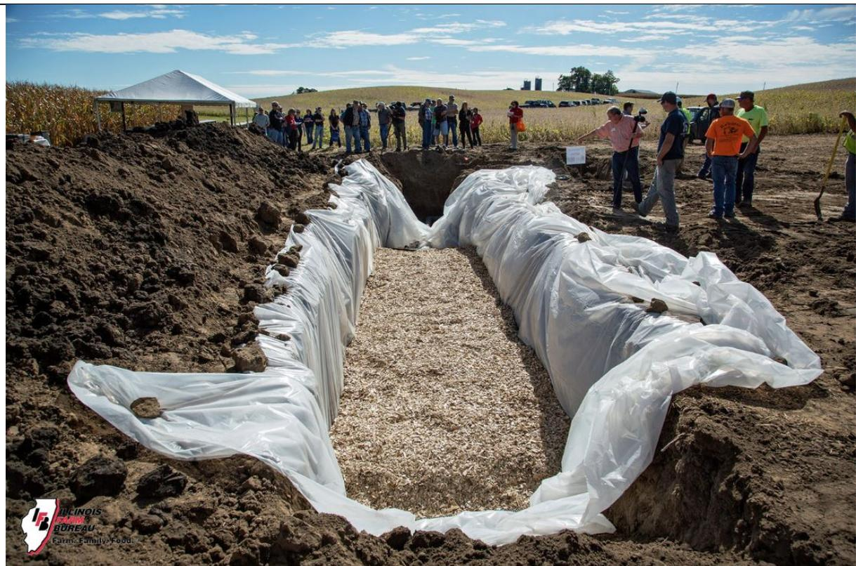
**Figure 9a:** Denitrifying bioreactor during construction on a farm in Illinois, USA. *Credit: Illinois Farm Bureau.*
