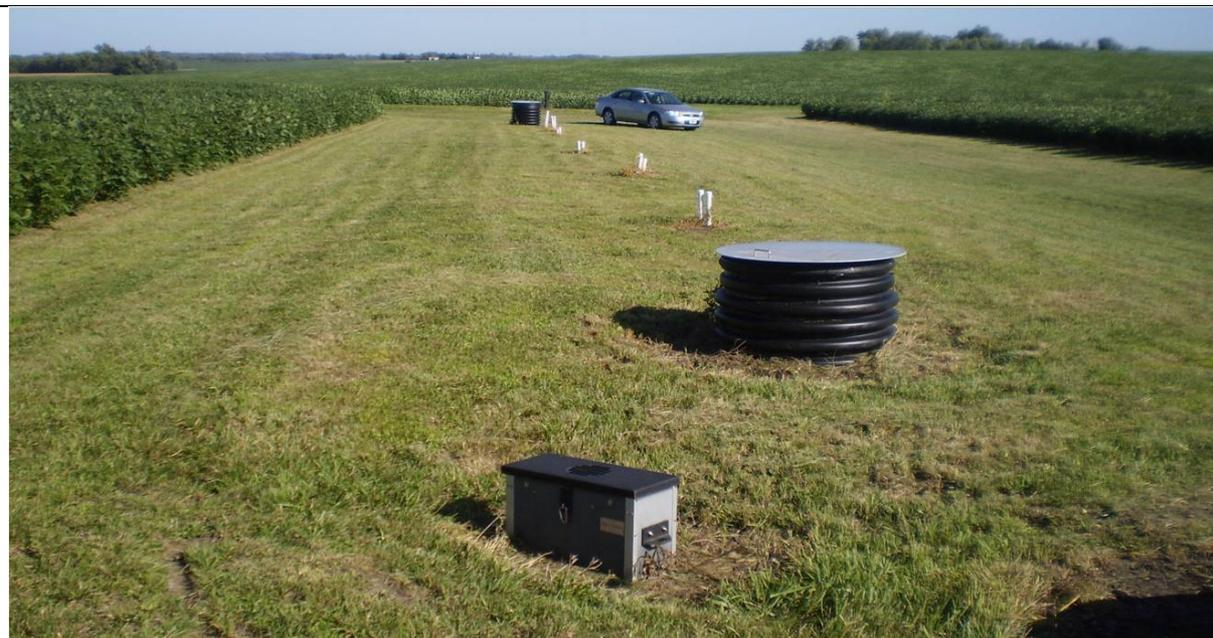
**Figure 9b:** Completed denitrifying bioreactor in Iowa, USA. The white pipes are water sample monitoring wells and dark gray rectangle is the inflow control structure. *Credit: L. Christianson.*
