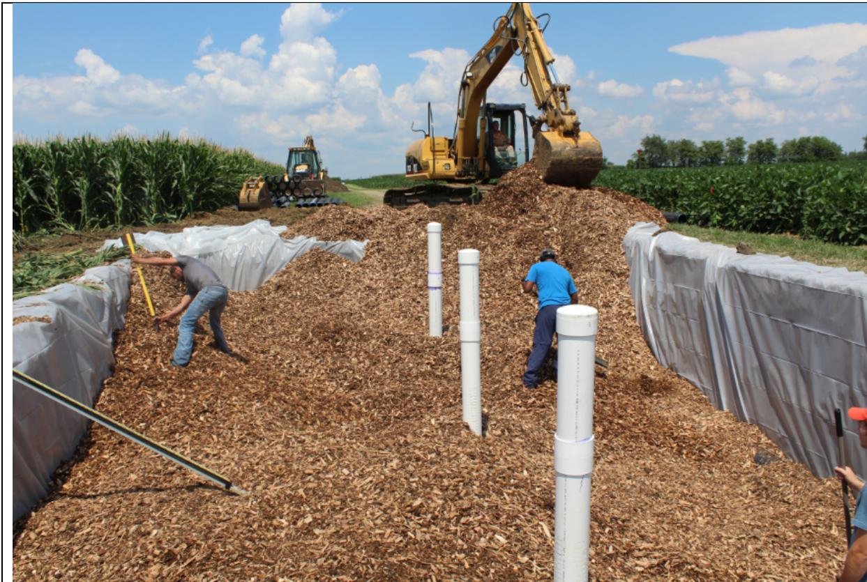
**Figure 6c:** Installation of monitoring points. Monmouth 2017: Denitrifying woodchip bioreactor installation in Illinois, USA with monitoring wells shown; Credit: J. Chandrasoma/UIUC.
