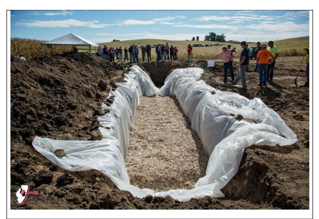
Figure 9a: Denitrifying bioreactor during construction on a farm in Illinois, USA. Credit: Illinois Farm Bureau.
