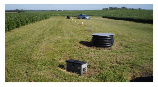
Figure 9b: Completed denitrifying bioreactor in Iowa, USA. The white pipes are water sample monitoring wells and dark gray rectangle is the inflow control structure. *Credit: L. Christianson.*
