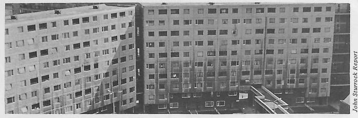
Liverpool: 1971, walls of compressed straw, floors of reinforced chipboard . . .
