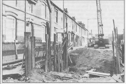
The Adderley Road trench. The houses on the left are all occupied. The metal supports for the sides of the trench were all pile driven into the ground.
