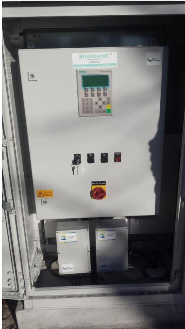
*Figure 8 Steinhardt control panel and EMS LMCS hardware installed in kiosk.*
