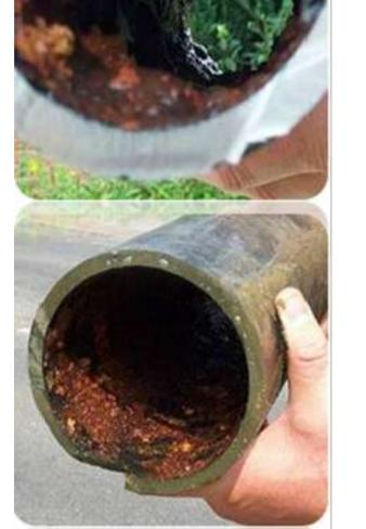
Fig. 1: Biofilm development within drinking water pipes.
